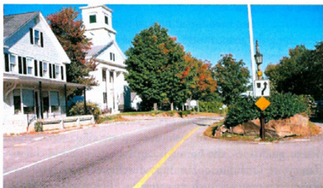
The historic town oval was restored to its original dimensions, returning its aesthetics and calming traffic by requiring drivers to pay closer attention as they navigate the channeled lanes.
