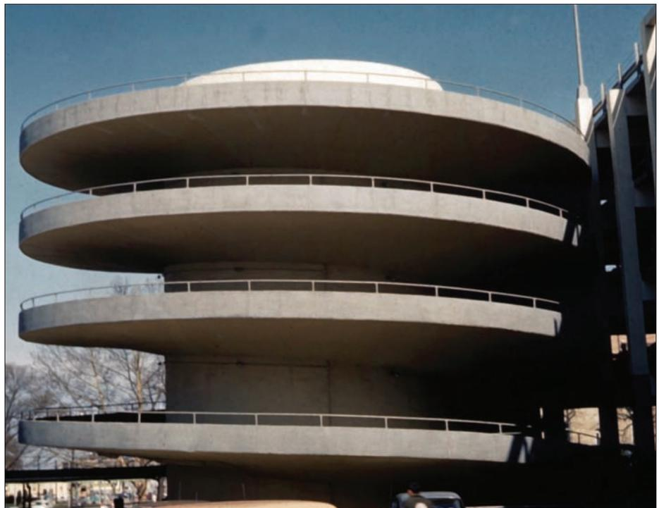
TOP: The first consideration in creating cost-effective parking is the size and shape of the site on which the facility is being developed, which impacts both the efficiency and layout of parking. ABOVE: Although spirals are efficient in handling the capacity, spiral ramps are generally very expensive to build.
