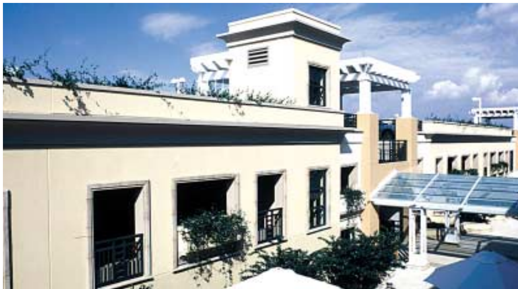
A living roof, which is essentially a large garden, reduces urban heat island effect and provides a nice public area for patrons.
