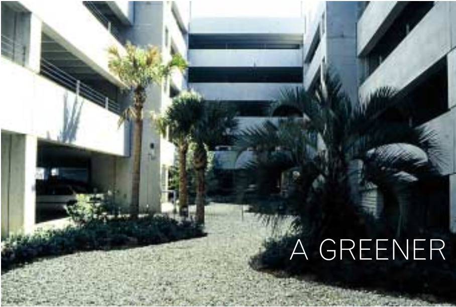
Landscaping can make any parking structure more attractive, while reducing urban heat island effect.
